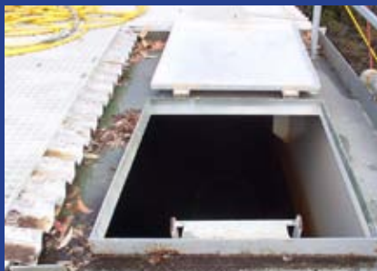
Entry hatch after
