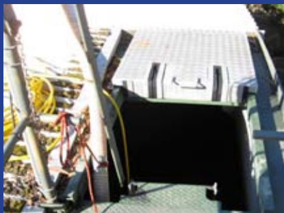
Entry hatch before
