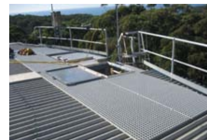
After platform renovation
