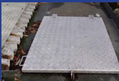
New entry hatch closed
