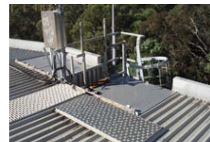
Before platform renovation
