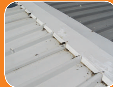
Ridge capping appears to be sealed.
