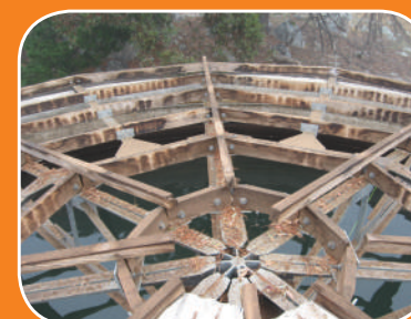
Centre pitched roof debris.
