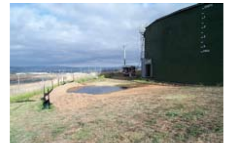
Waste water disposal to coffer dam
