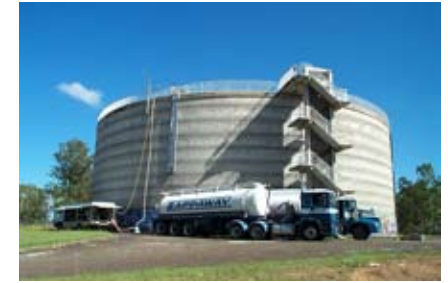
Waste water disposal to tanker
