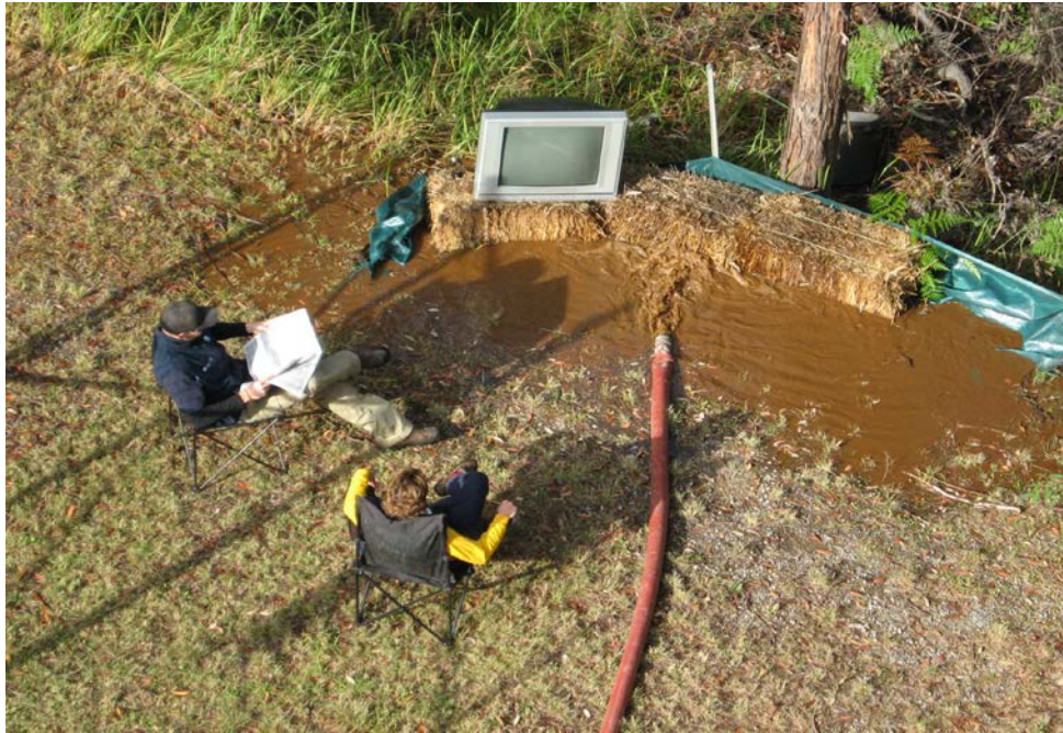
Figure 1 Hay Bale Cofferdam
