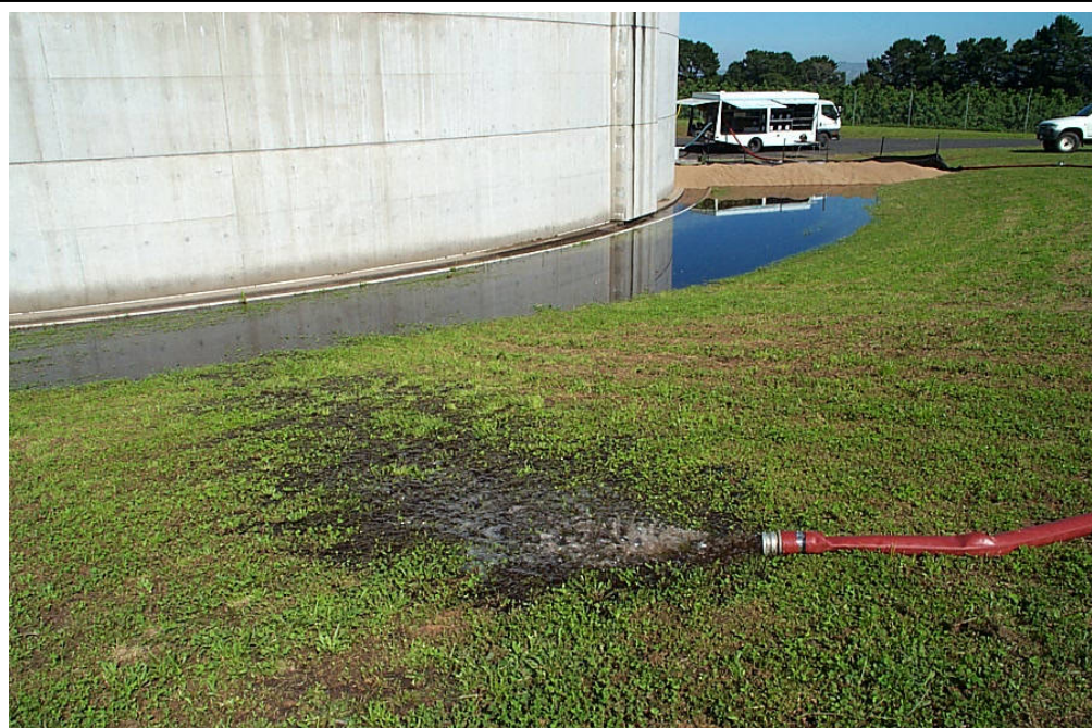
Figure 4 Tank Wall Coffor Dam using coarse sand
