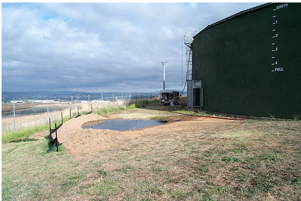
Figure 2 Course Sand Cofferdam
