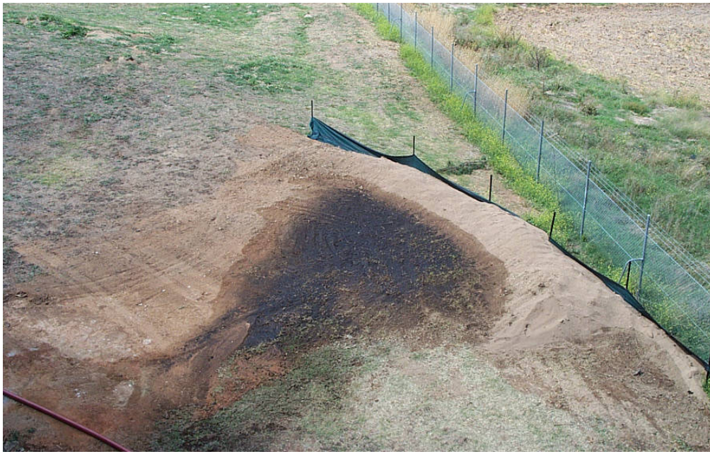
Figure 3 Course Sand Coffor Dam after water has soaked away
