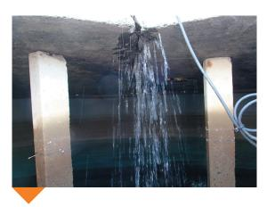
The first method is using a clean bucket and rope to obtain water from the tank and then pour it around any areas that should be sealed, such as platform edges, hatch frames and any fixtures set onto the roof area. And then look (and listen) inside the tank to see or hear any water ingress.
