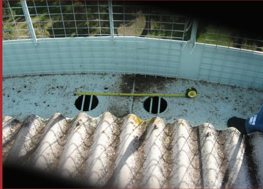
**Most storage tanks have been roofed to maintain water quality, and at first glance this is a marked improvement upon the previous uncovered storages. However, roof areas can hide a multitude of contamination problems that are not obvious at first.**
