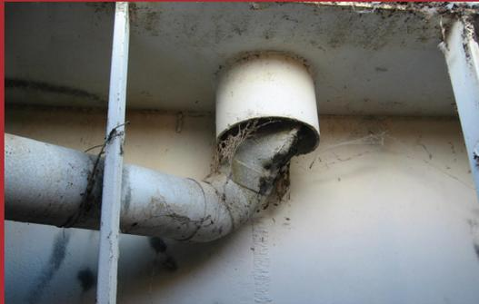
Faulty drainage points are the largest contributors to 'unseen' contamination – often the whole roof area keeps on draining back into the tank, along with the surface contaminants that have accumulated upon it.
