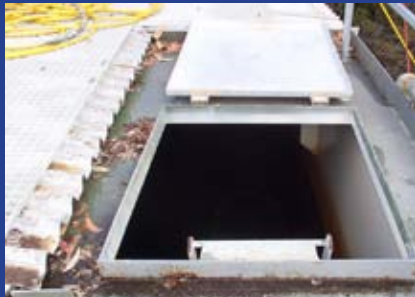
Entry hatch after
