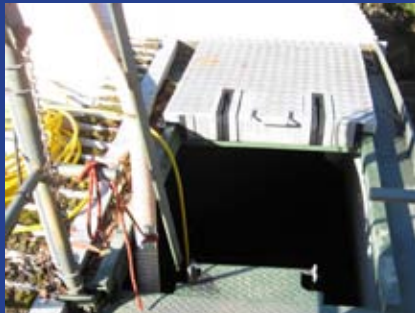
Entry hatch before
