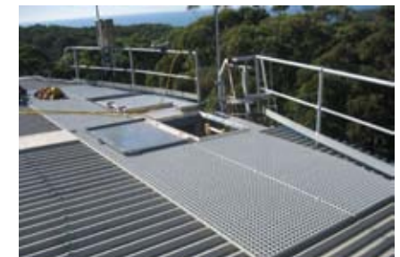
After platform renovation
