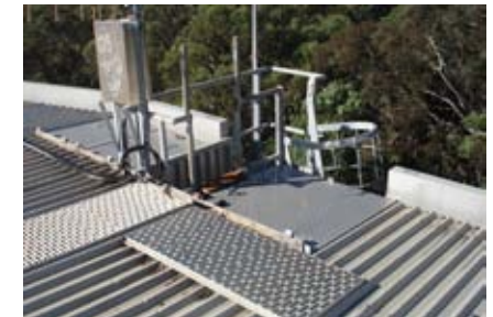
Before platform renovation
