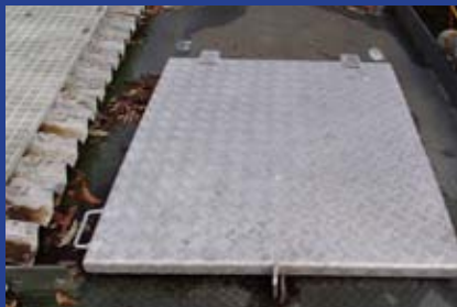
New entry hatch closed
