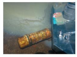
The presence of heavily corroded internal ladder systems and overflow pipework, along with excessive sediment loadings are also important to identify, as they will be impacting disinfection residuals within the storage (Barrier 3).
