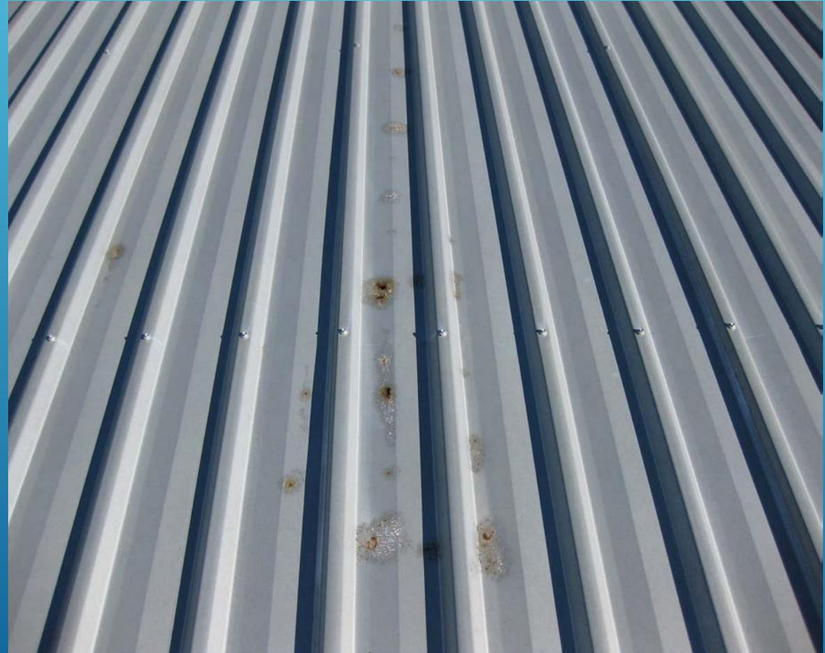
**Number 4:** Using roof framing materials that are not suitable for hot, moist and gaseous conditions. Zincalume coated purlins and rafters have a short life span in these situations and they also deteriorate quickly when roof screws puncture the surface coating.
