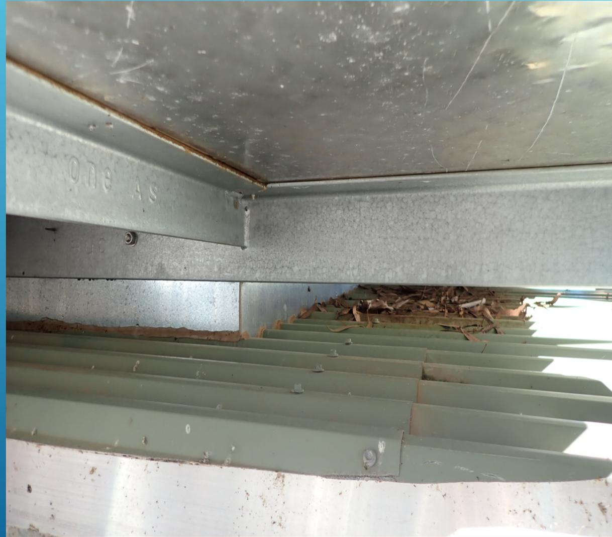
The worst platform outcome identified to date! A new platform was constructed over the top of the existing one, which was partially removed, leaving a large unsealed area leading directly into the tank.
