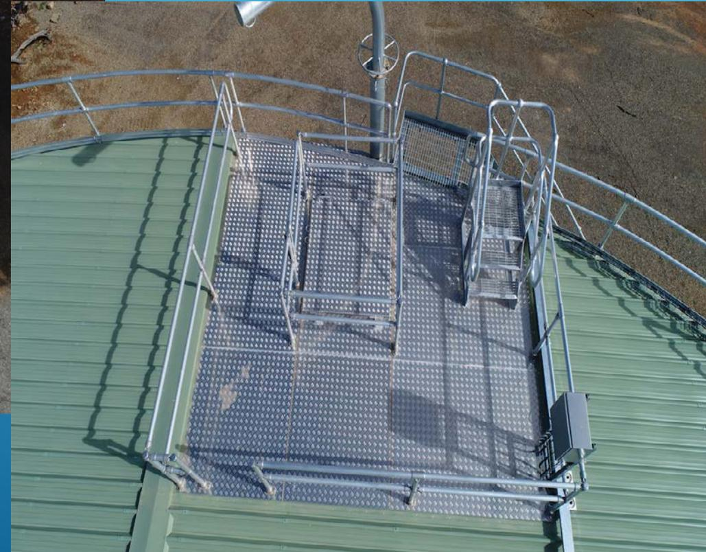
There are too many unnecessary handrails around the entry hatch and platform areas.
