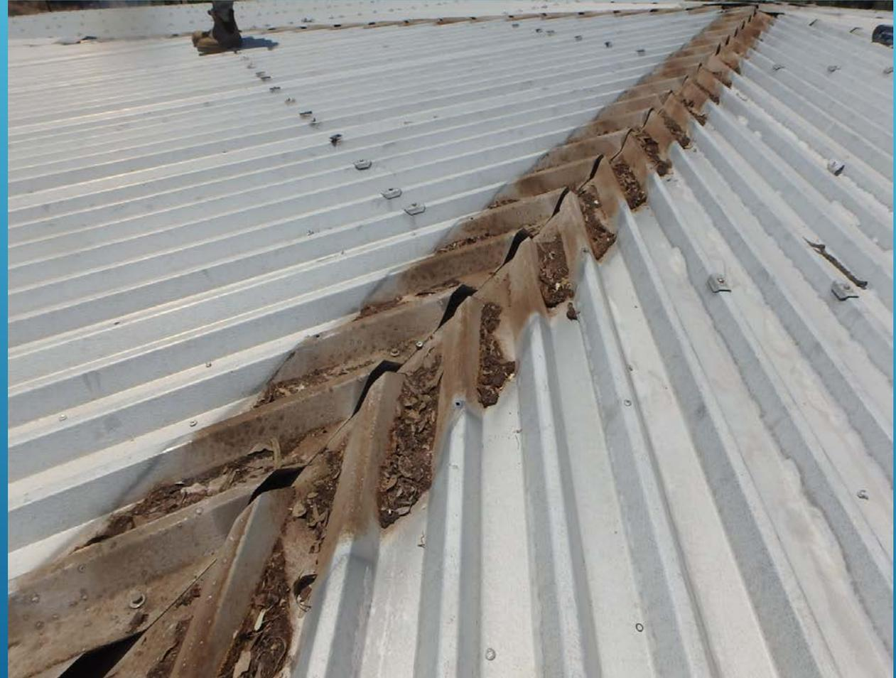
**Number 3:** Placing safety mesh under the roof sheets to comply with OH&S during construction. This material is usually the cheapest available and corrodes quickly, causing the roof sheets to fail and then dropping the debris down into the tank and making regular cleaning of the floor difficult. In a factory situation, there would have been a layer of insulation between the mesh and the roof sheets.
