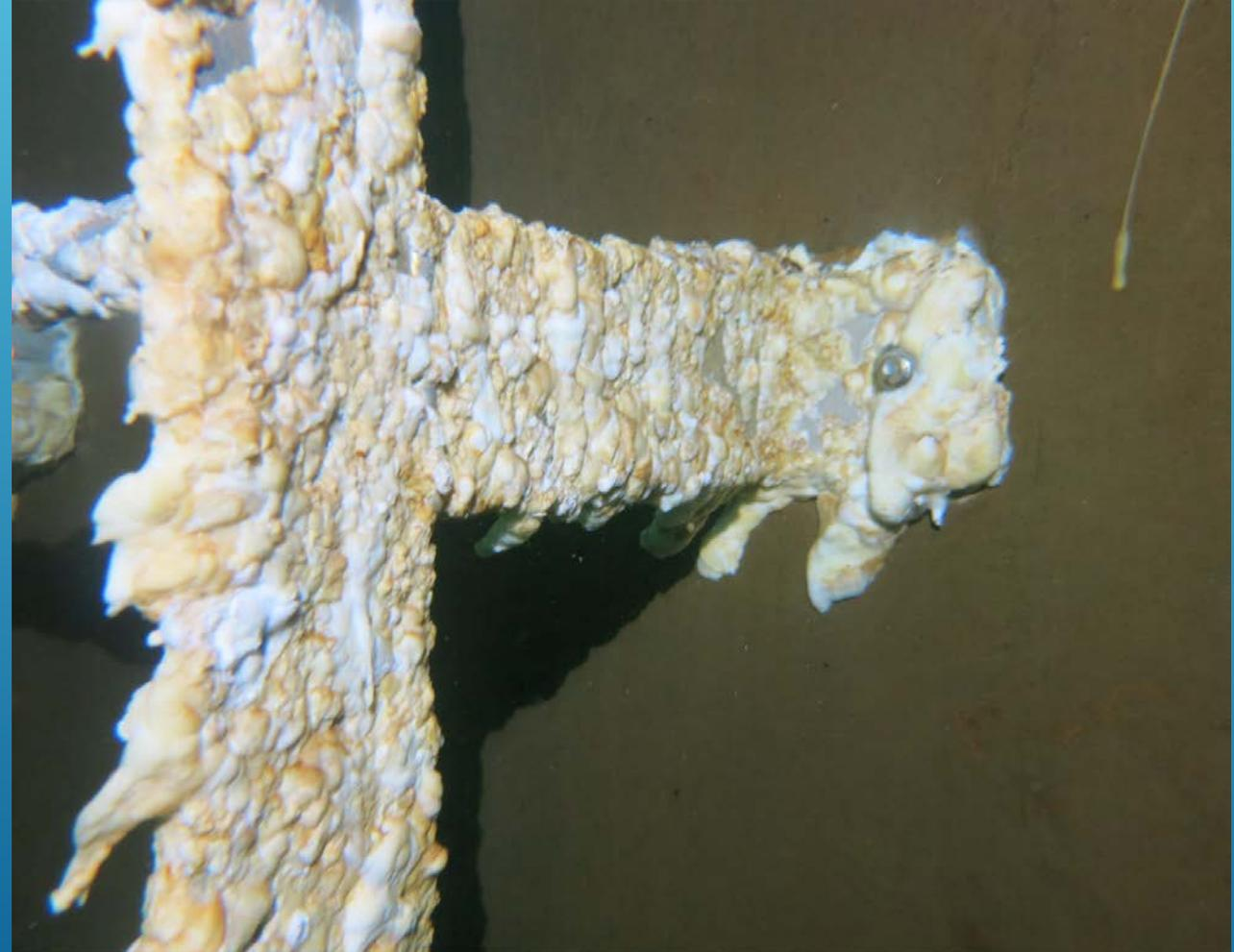
**Number 9:** Not thinking about how internal pipework will affect the stored water quality. Inlets placed next to outlets lead to short circuiting issues. Outlets close to the floor allow sediments to be drawn into the downstream reticulation system. Scours not being fitted in the lowest area of the wall or floor will not allow for effective draining of the tank.
