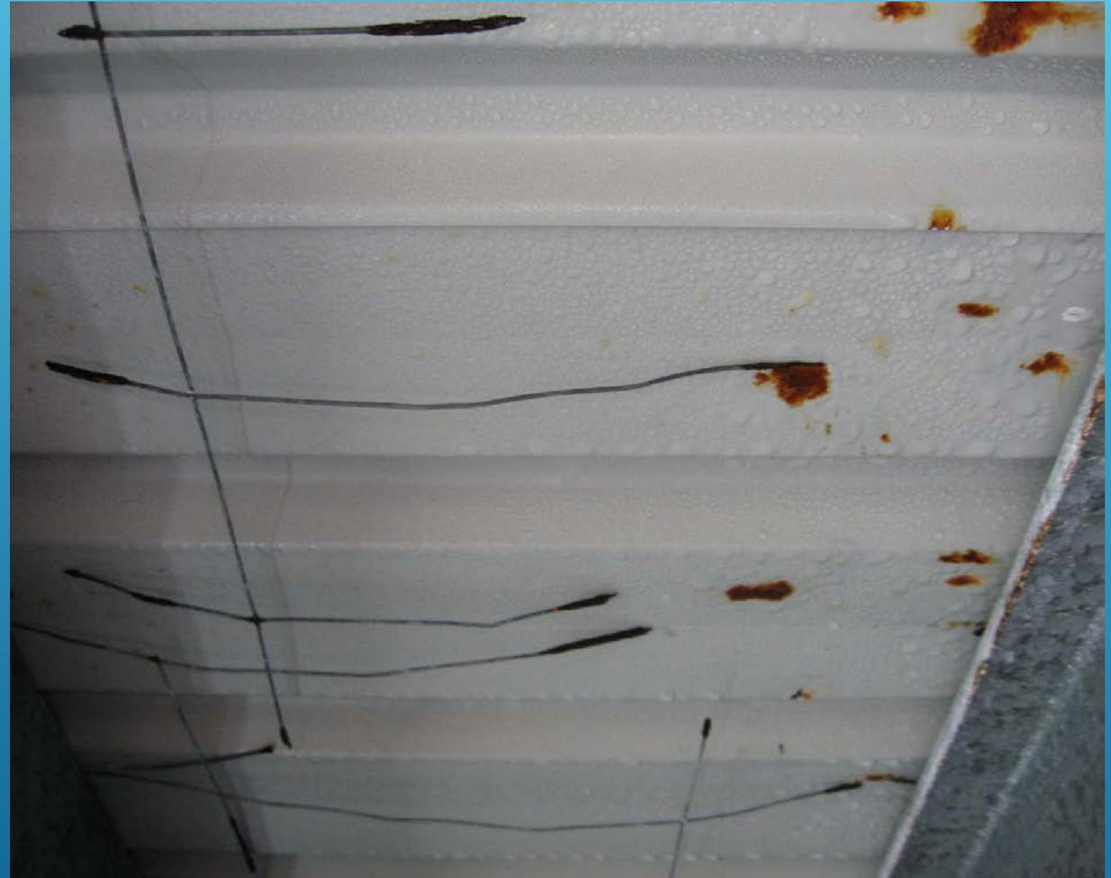
The corroded safety mesh breaks away and drops down onto the floor area, making effective tank cleaning a near impossible task. It also corrodes the roof sheets from the underside, leading to structural failure and an unsealed roof surface.
