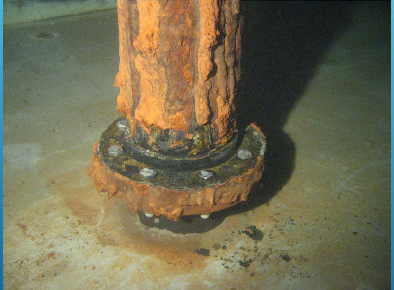
Aluminum posts corrode quickly in some waters, depending on pH levels. The SS bolts also contribute to the aluminum deteriorating. Another factor is the posts not being isolated from the floor fixings and roof framing, as they quickly become an anode to protect the reinforcing steel in the concrete walls and floor.
