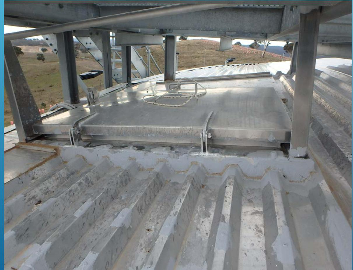
This platform sits just above the roof area, which creates a safe habitat for birds to nest below it and for leaf debris to build up and damage the roof sheets. The hatch frame is also only sealed onto the roof sheet edges with mastic and there is no easy access to repair it when it deteriorates and allows the localized contaminants to enter into the tank.
