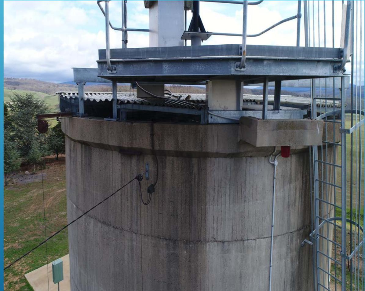
The entry hatch cover was then made up as an extended section and dropped down into the open roof hole. While it wasn't sealed onto the new platform area around the edges, below the platform was a far worse sealing issue!
