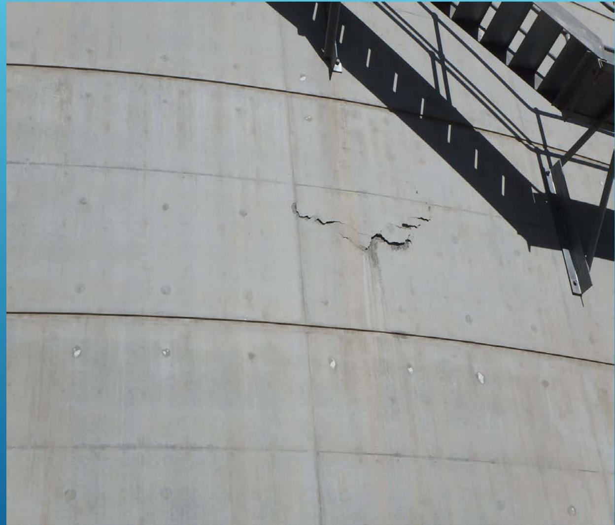
**AND...Number 11:** Having no understanding of short and longer-term maintenance requirements. Just because a tank is new, does not mean it will require no maintenance. Good external access for EWPs, cranes, service vehicles and larger trucks is often necessary for roof repairs after storm events. Steel tanks will need to be recoated after 30 years of service, so a good-sized flat area for parking the necessary heavy equipment should be factored in.
