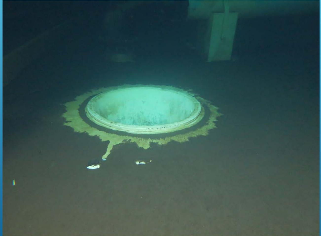
The scour penetration is 120mm up off the floor area, which makes it impossible to fully drain the tank.
