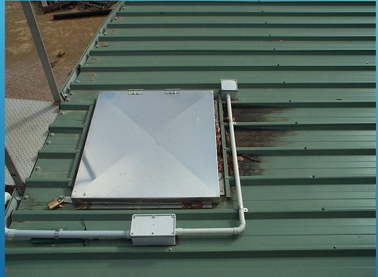
This entry hatch cover sits directly on top of the roof sheets with no frame or sealing mechanism in place around the edges. The internal ladder stiles extend through the unsealed hatch cover. The tank also has a significant amount of local bird activity and their faecal contamination is entering directly into the stored water.
