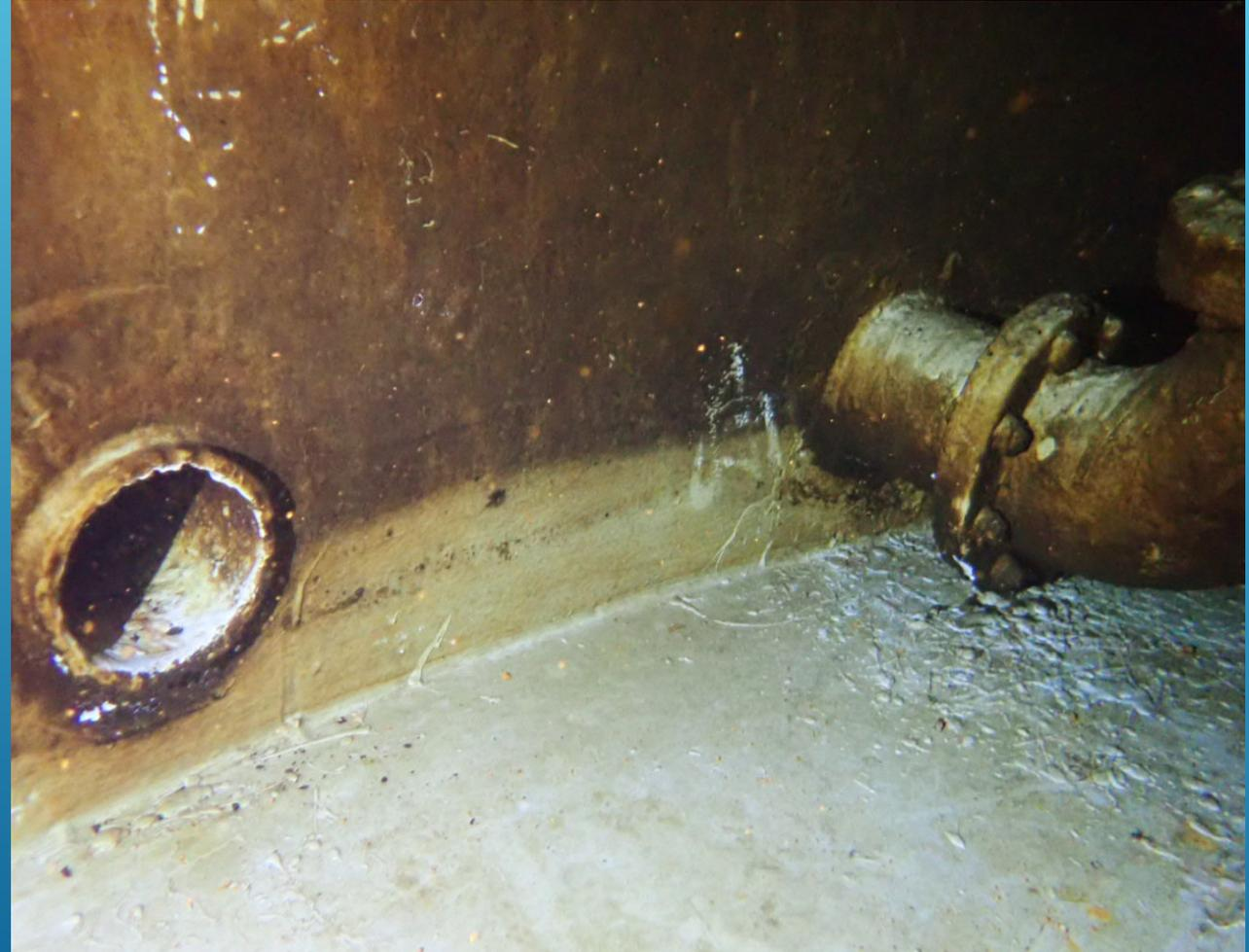
The scour penetration is 80mm up off the floor area, which makes it impossible to fully drain the tank. This is a new tank, so cut and paste must have occurred in the design.
