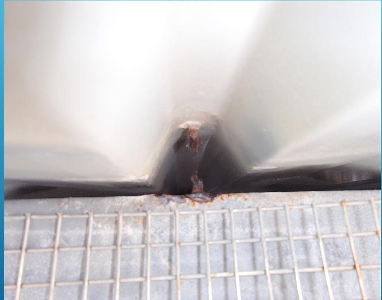
**No7:** Aluminum roof framing that is not securely fixed. While aluminum is a good corrosion resistant material, it has a lot of flexing movement and will loosen off the fixing bolts unless nylock type nuts are used. Being a softer material to steel, extra thickness is also required for edge flashings, as fixing screws are prone to pulling out in windy conditions.
