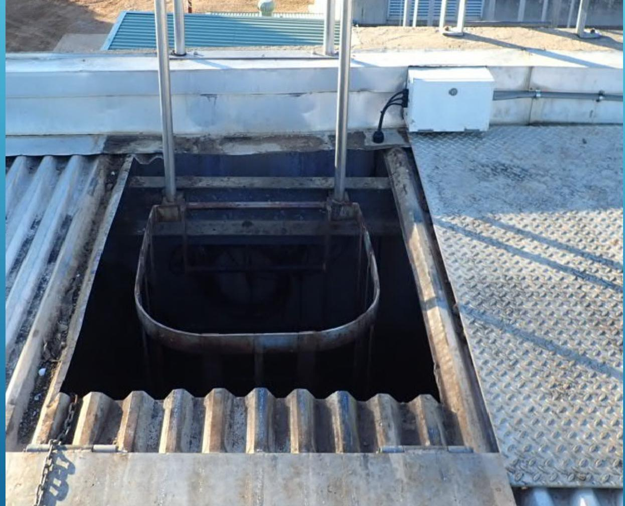
Flashings on the edge of roof areas prevent rain water from draining off and ridge cap flashings are difficult to seal and allow all sorts of debris, bird nesting and vermin entry to occur.
