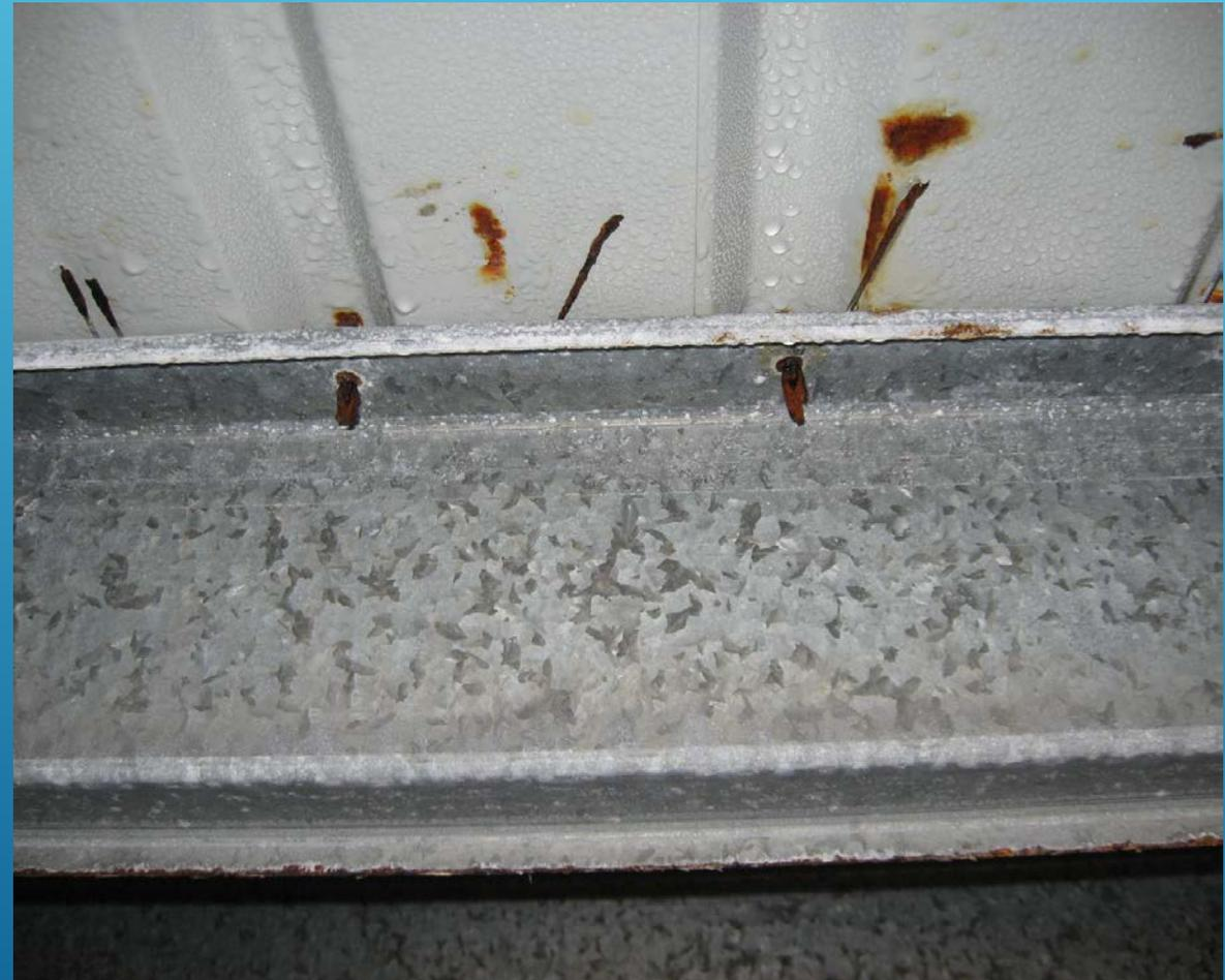
Cheap roof screws corrode away in warm, moist conditions. The roof sheets are then left unsecured as the image on the RHS indicates. Only category 4 Buildex type screws should be used in these conditions.
