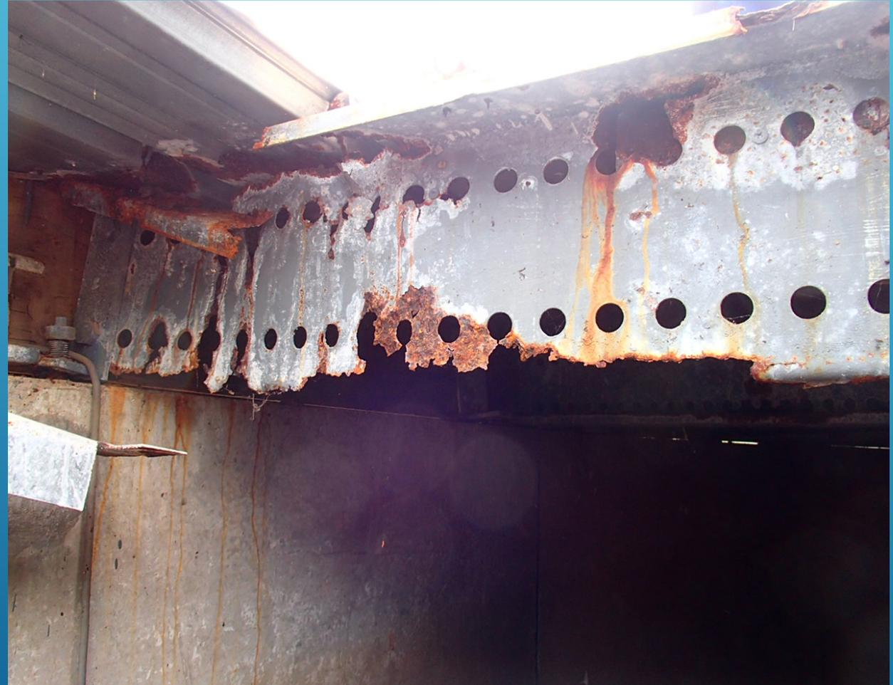
Zincalume purlins and rafters corrode heavily in warm, moist conditions. They are also quick to break down when immersed, if the tank water level settings are not adjusted correctly as the image on the RHS indicates
