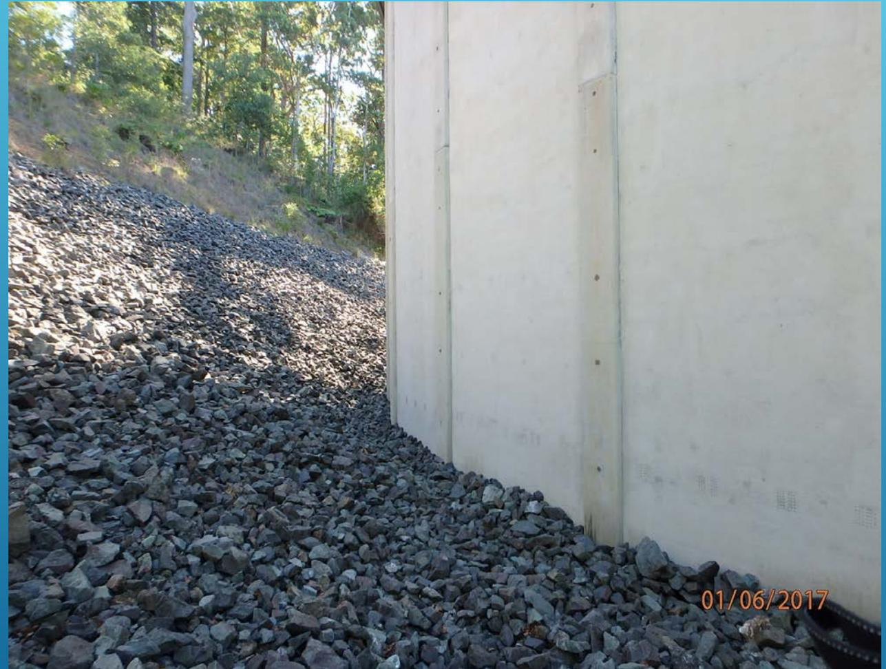
The backfilling has caused the walls on this tank to spall in the middle areas, after three years in service.
