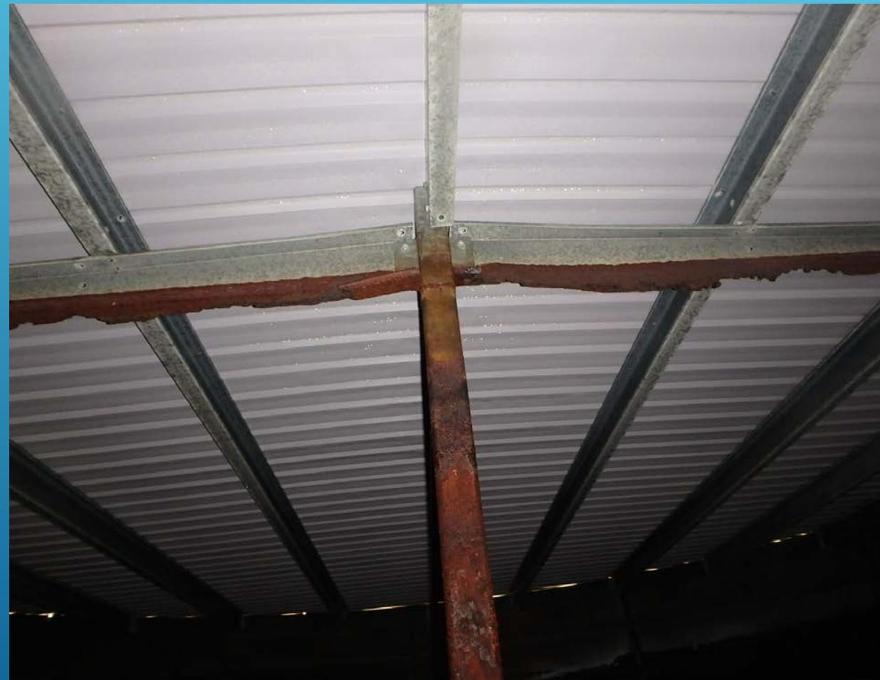
**Number 5:** Roof screws that are not rated for marine or extreme conditions. The roofing contractor often uses the cheapest type of screw to reduce costs, but corrosion failures are now occurring under five years in some environments.
