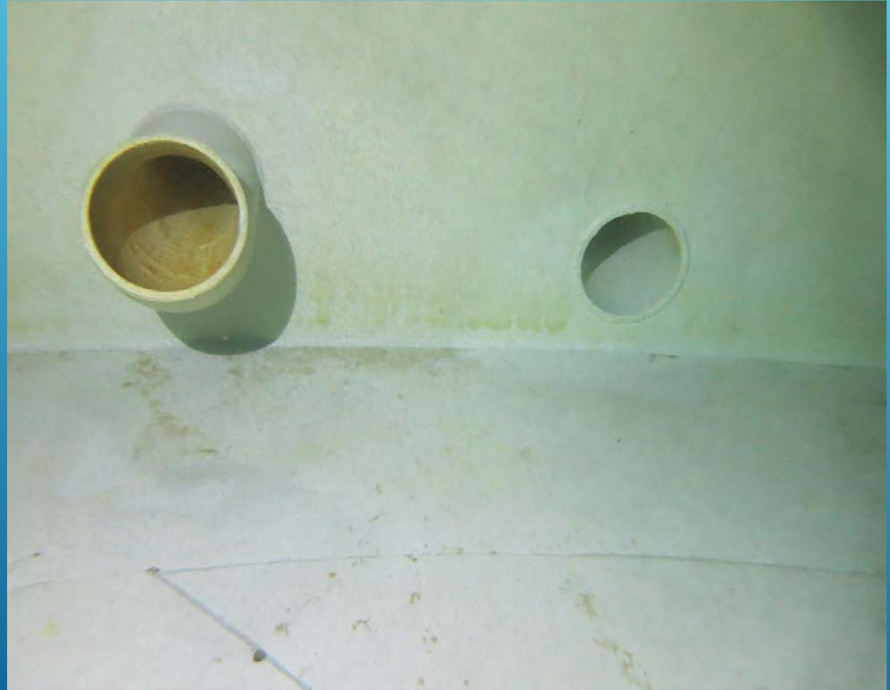
**Number 10:** Building a tank whose walls are designed to move in and out under pressure and then the client back-filling directly against those walls, to save money on a retaining wall. This leads to significant structural damage and a complete failure of the tank in some circumstances.
