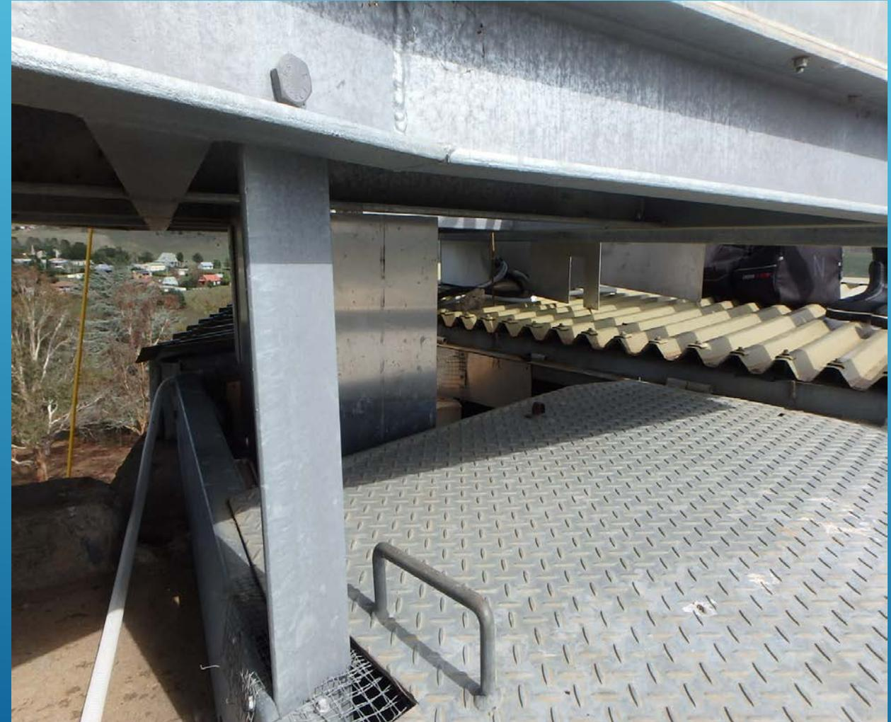
Entry hatches mounted too far off the wall, so that ladder supports have to be extended to accommodate the excessive distance.
